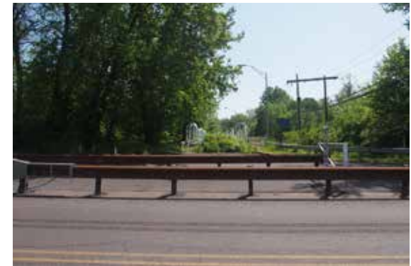
The newly aligned Keim Street will create a 4-way intersection at Industrial Highway, lining up with the new Keim Street Bridge across the Schuylkill River.
