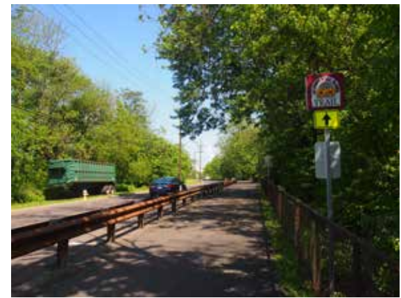
Bicyclist exiting Keim Street onto Industrial Highway must ride in the travel lanes since there is no opening in the guide rail along the Schuylkill River Trail.
