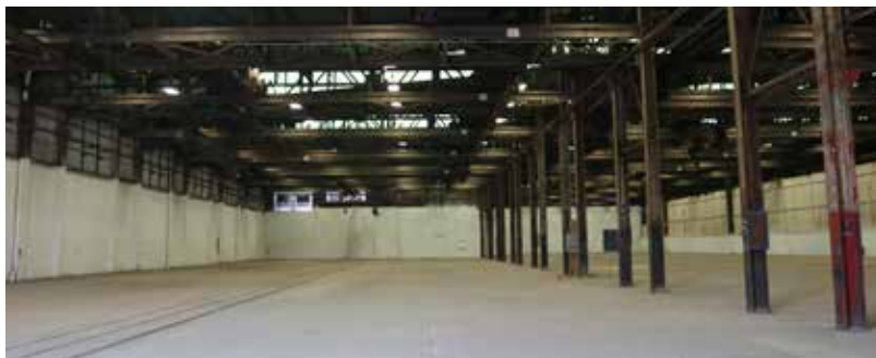
Interior of a warehouse bay at the Pottstown Industrial Complex
