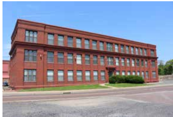
The historic office building at 200 Keim Street.
