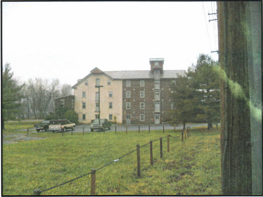
Adjacent Land Use (West of Subject Site)
