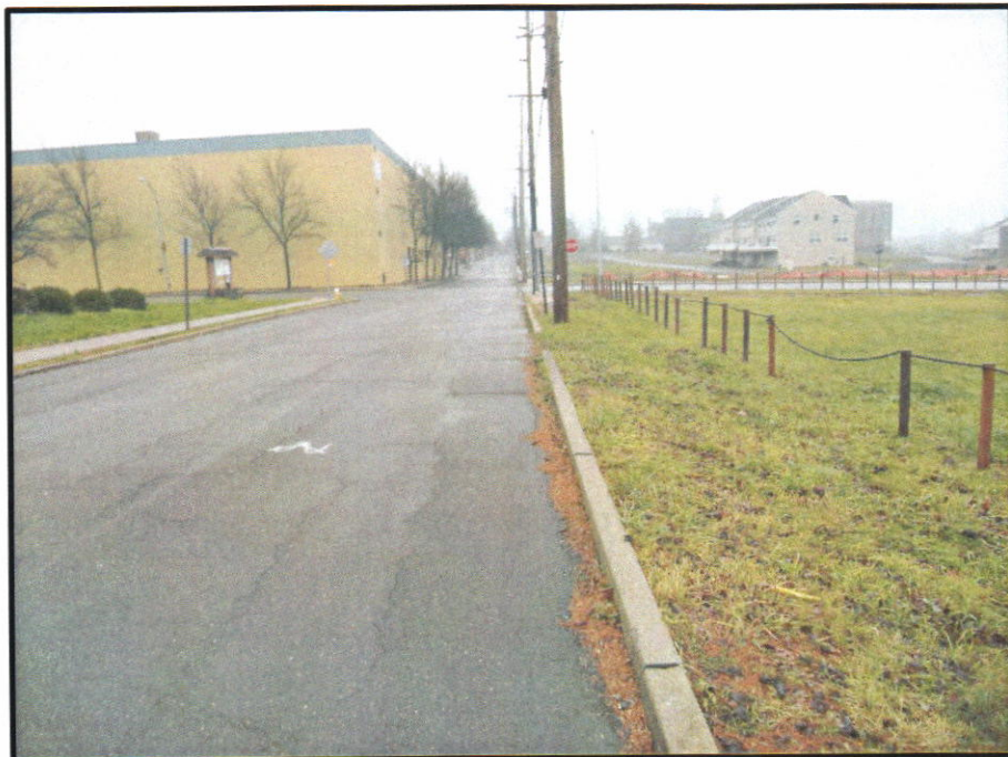
South Street Facing West
