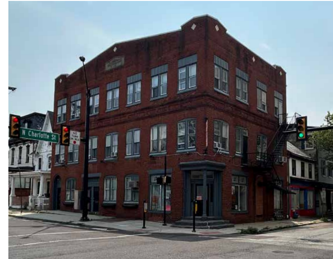
300 King Street is an example of a very healthy facade.
