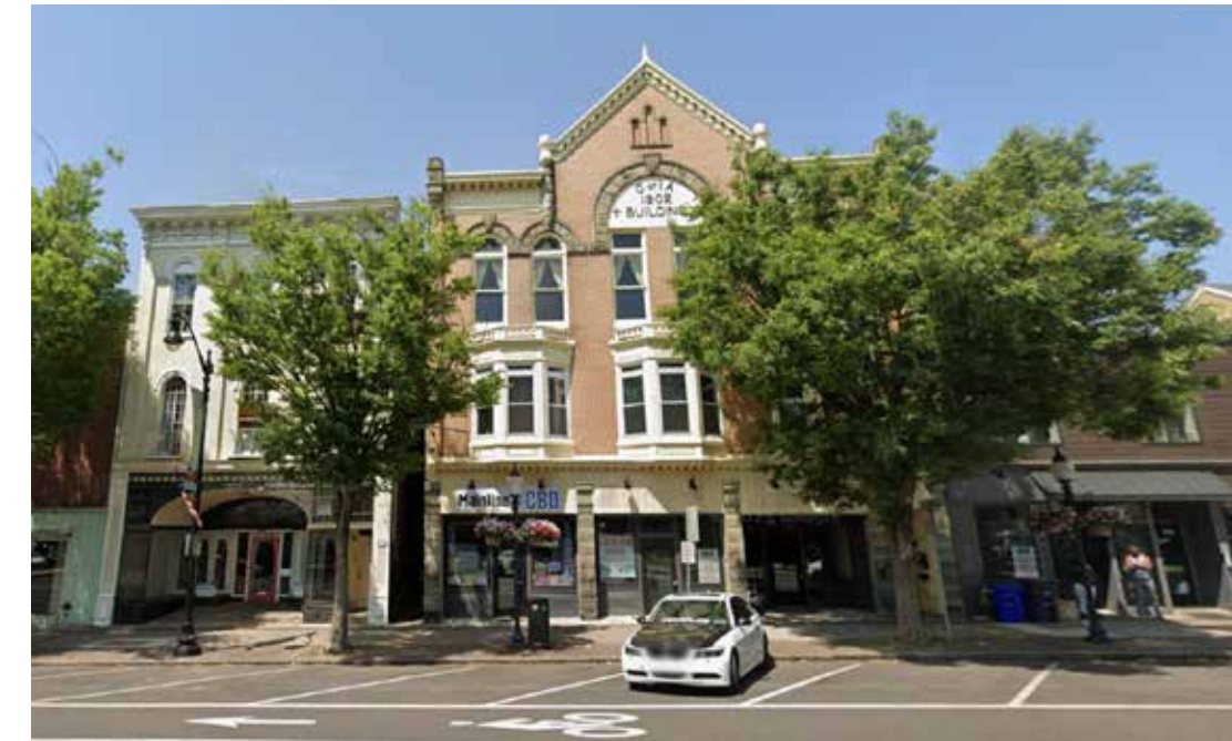
309 E High Street is an example of a very healthy facade.
