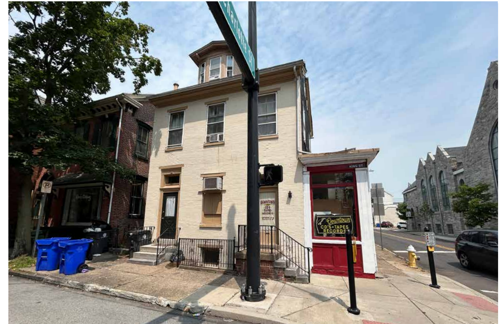
51 North Charlotte Street is an example of a very healthy facade.
