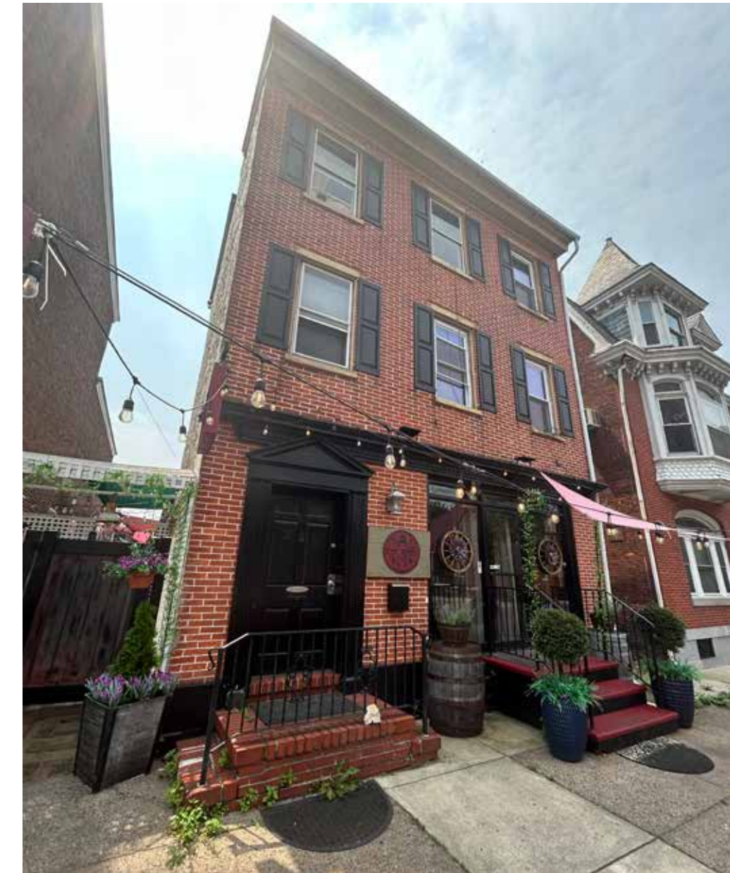
232 King Street is an example of a very healthy facade.
